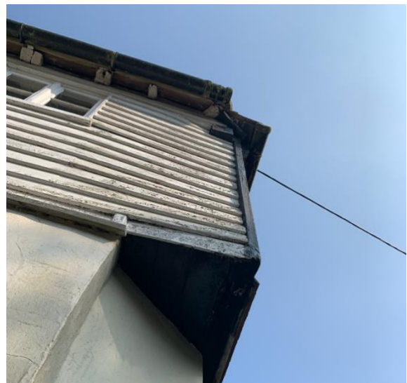
Jettied corner with missing dragon beam
